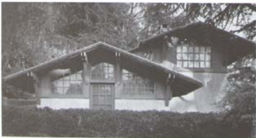
Bottom: Maybeck's Mathewson House, Berkeley (1916)
