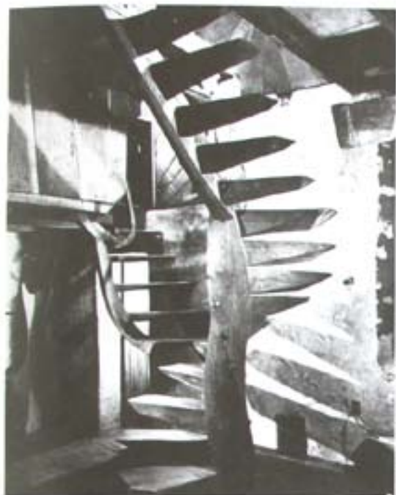
Left: The spiraling oak-trunk stair in Wharton Esherick's studio; the sculptor said of it: "No one will fall down this stair. It's too dangerous."
